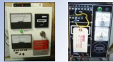
Impressed Current Rectifiers
