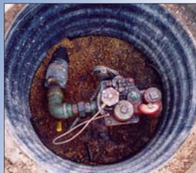
No Corrosion Issue
